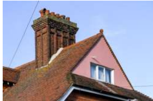
Photo 18 Chimney detail (Photo 17)
