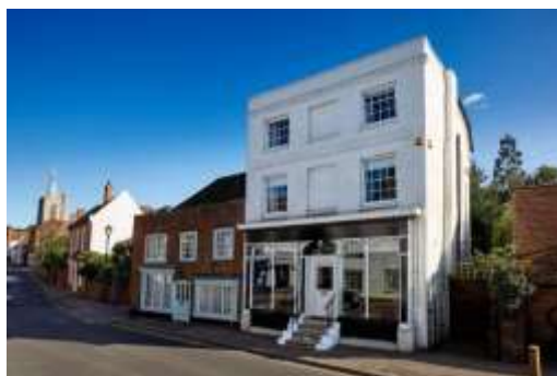
Photo 31 South side of The Street
