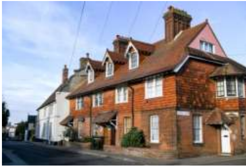
Photo 17 The Street corner with Queens Road
