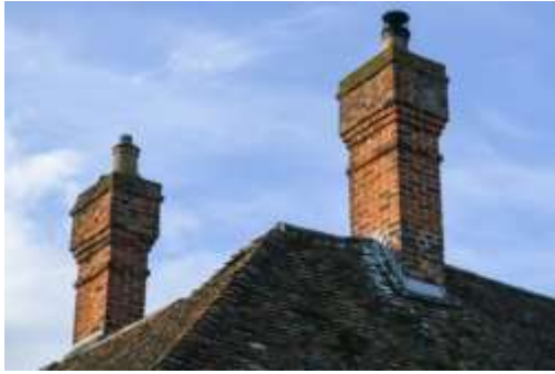
Photo 15 Chimney style Tudor Cottage (Photo 13)
