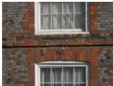
String course brickwork
