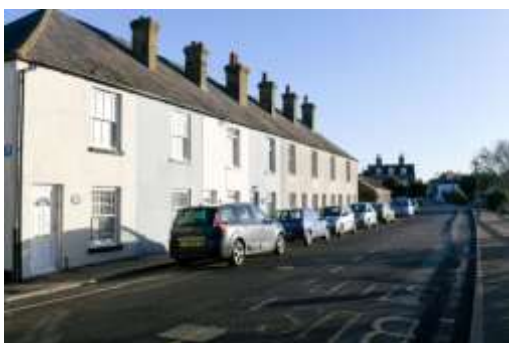
Photo 3 Mid-19 th century terrace cottages looking to Street End house
