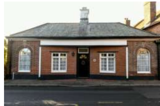
Photo 10 Shop converted to domestic use (opposite Vine House Photo 7)
