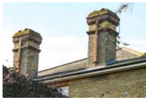
Photo 40 – chimney detail (of 5 The Street)
