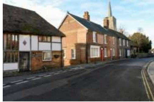
Photo 16 Terrace cottages beside St Nicholas Church
