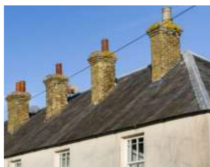
Photo 4 Chimney style on the terrace
