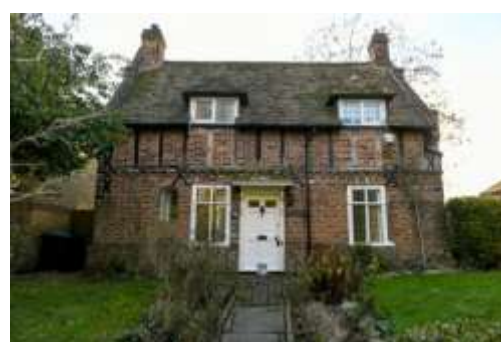
Photo 38 7 The Street (Yeoman Cottage) Grade II 1624
