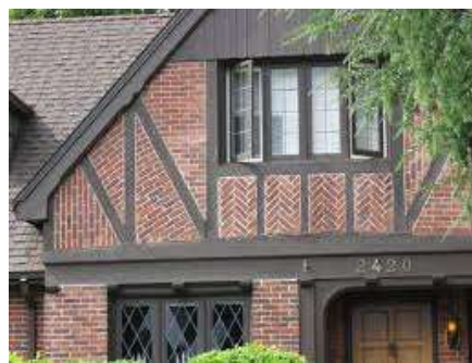
Brick noggin, herringbone brick
